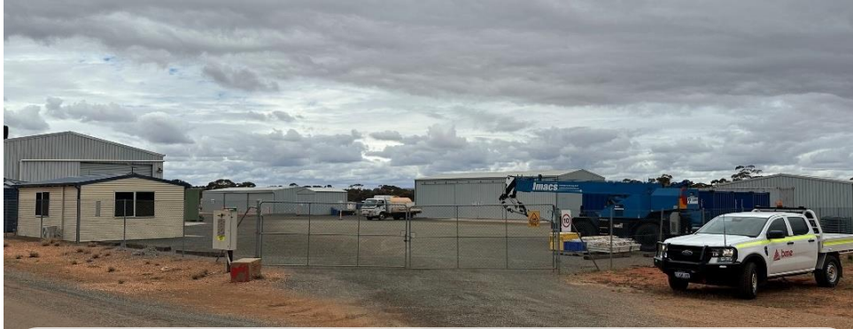
Kalgoorlie Government Reserve, Western Australia – AXXIS Plant
