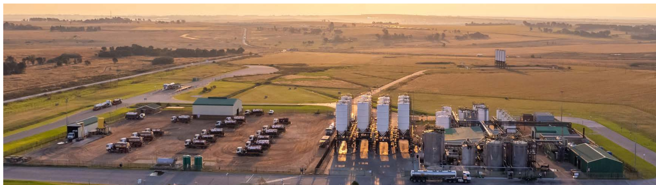
Dryden plant, BME, Delmas
