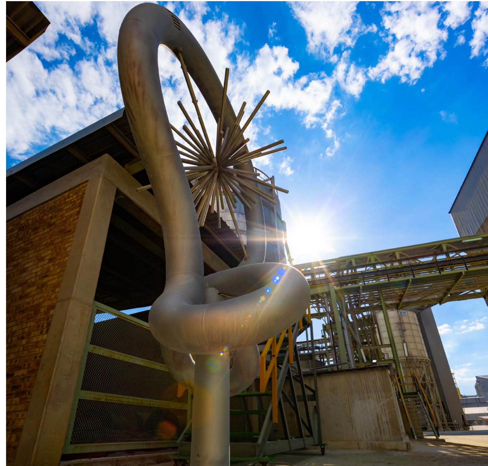
Nitrophos 2 plant, Sasolburg
